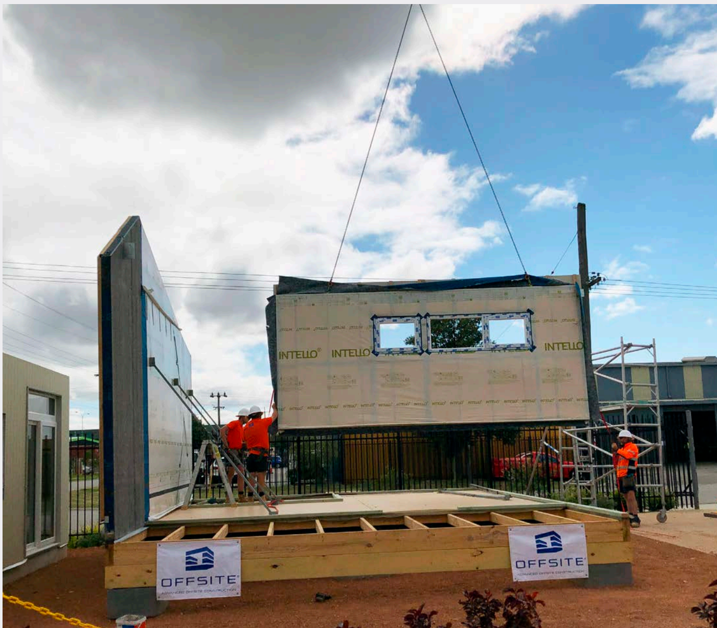
The units were assembled from prefabricated panels, making for rapid assembly on-site.
